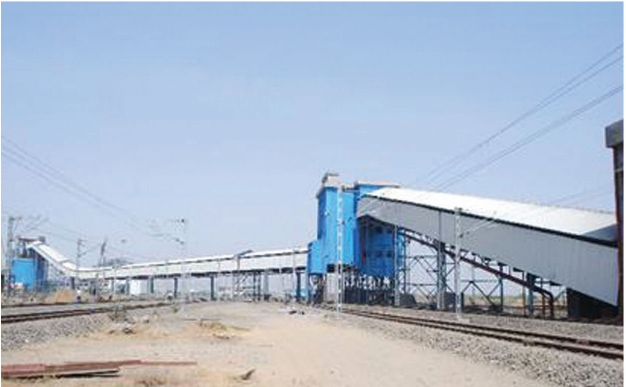
Bhusaval 4 Coal Conveyor Belt
