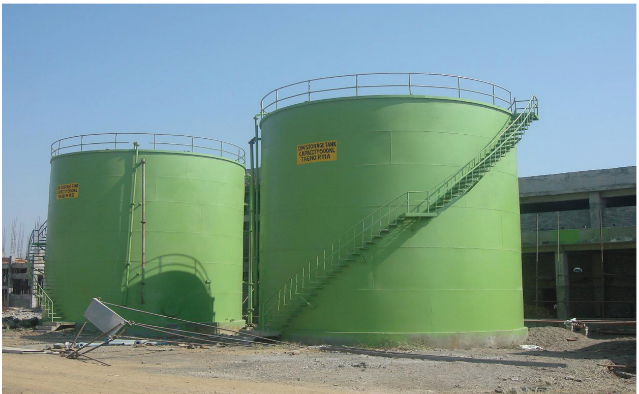
Parli Demineralisation Water Tank
