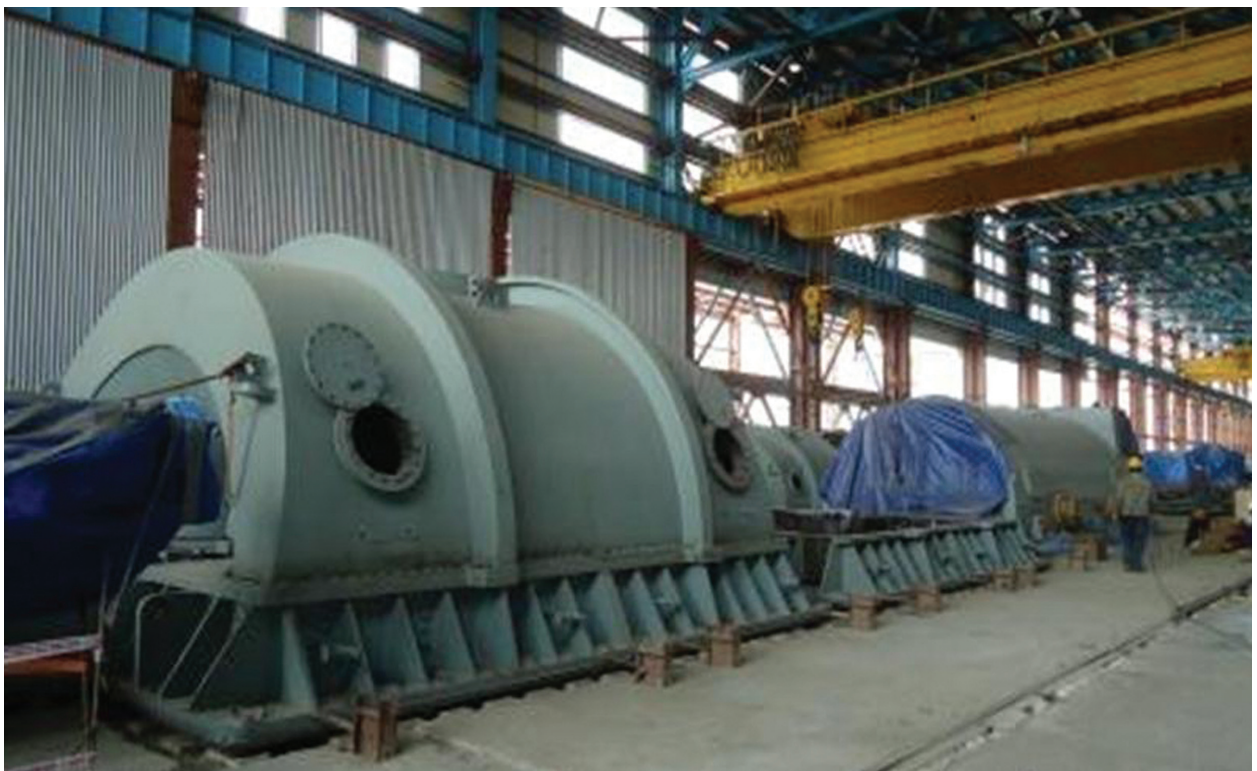
Koradi Turbine Unit Area
