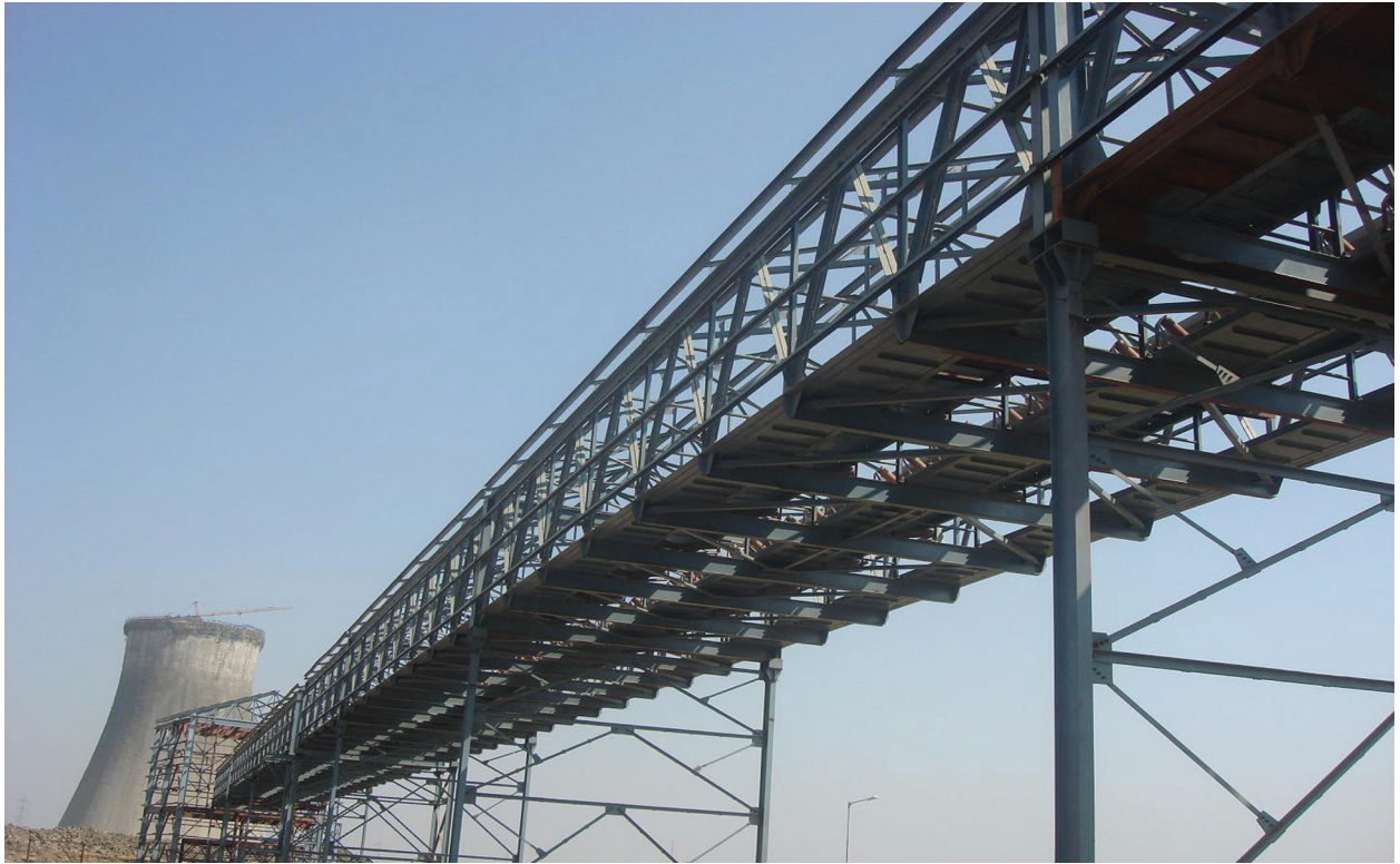
Parli Conveyor structure
