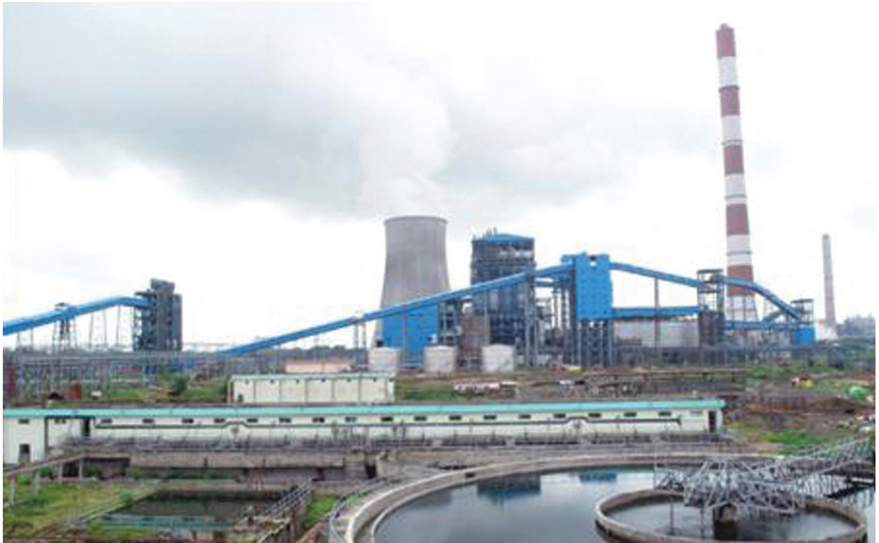
Khaperkheda Project view
